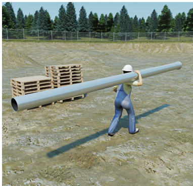
Pipes can often be handled by one man alone. However, please observe national guidelines on manual handling.
