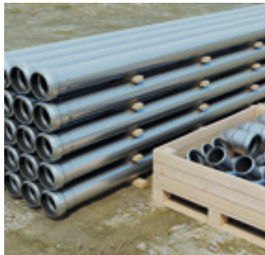
Pipe bundles and loose pipes should be stored on a flat surface and supported so that the pipes do not rest on their sockets.
