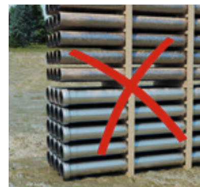
Do not store the pipes so that they come into contact with carbon steel which can leave traces of corrosion on stainless steel.
