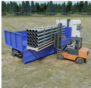
Pipes and fittings should be unloaded by forklift, alternatively by crane.
